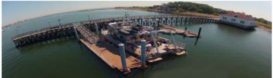
SBNMS pier and marine operations center
